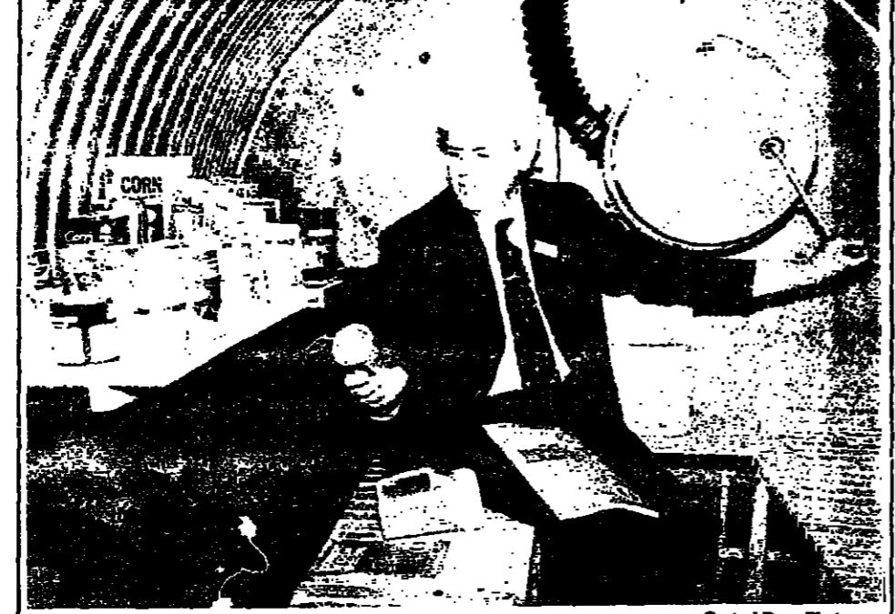
NUCLEAR SHELTERS: Domestic nuclear shelters are now being marketed in the West to provide protection against the effects of nuclear explosions. Picture shows the interior of a do-it-yourself type of shelter with an air intake pump and supplies of food reckoned to be sufficient for one adult for two weeks. These include canned foodstuffs.
